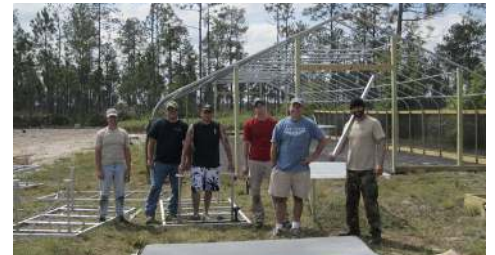
(Above) Adam and a team building the greenhouse.
